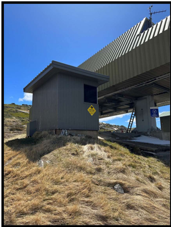
Figure 5 – View of the eastern elevation of the existing hut in summer when viewed from downslope. The hut is located on a filled mound to ensure it is at the correct height for the chairlift in winter.
